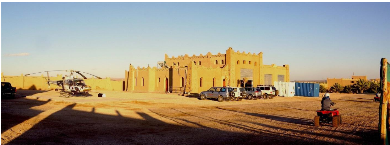
Figure 8 - The Ibn Battuta Field Facility
