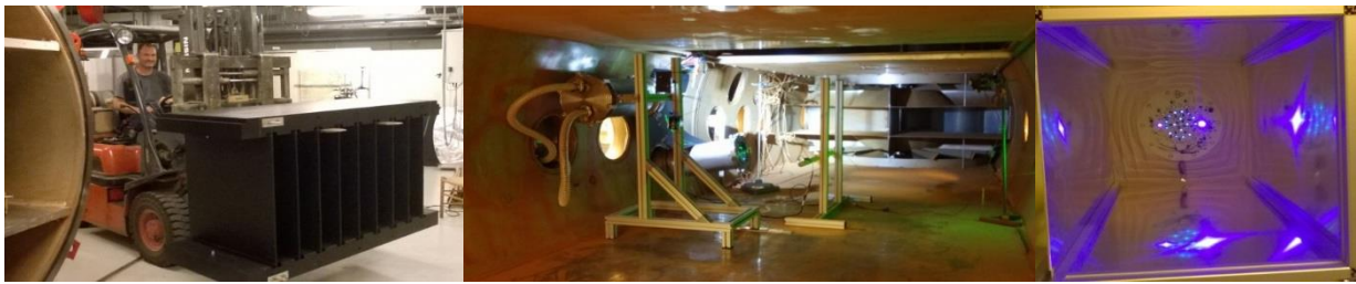
Figure 24 - Installation of the Particle Image Velocimetry at the Wind tunnel
